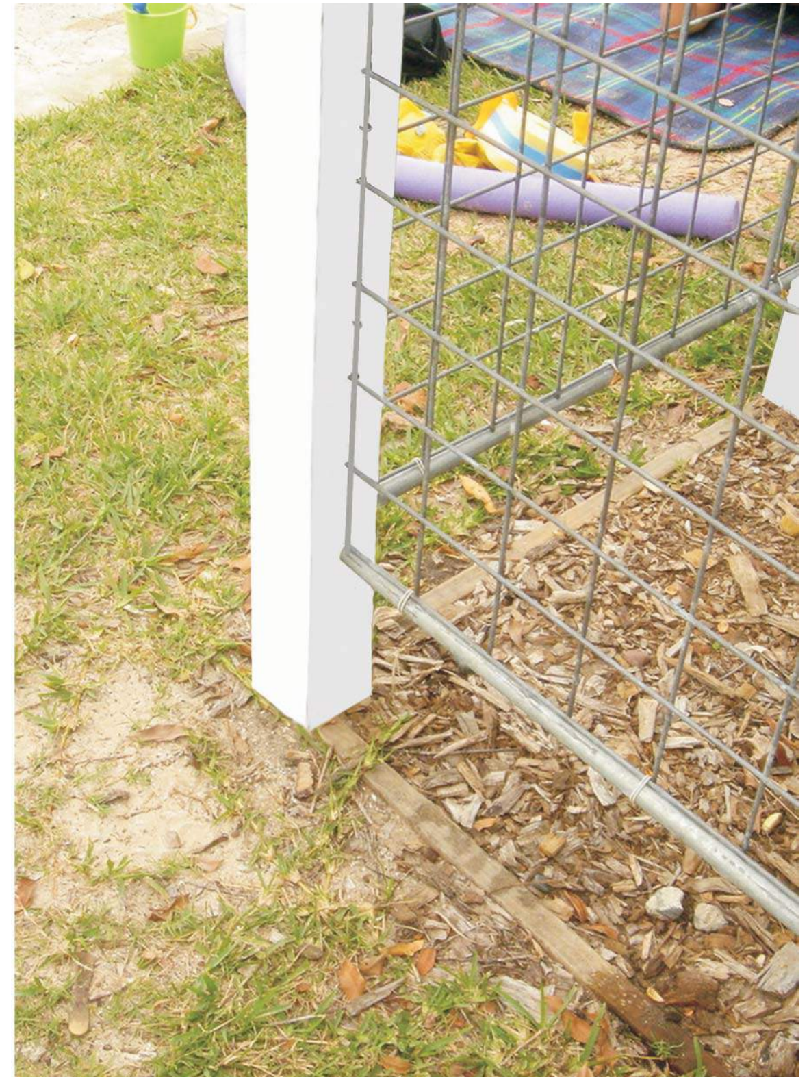
Proposed new tree barriers around street trees will have square white timber posts with wire infills .
